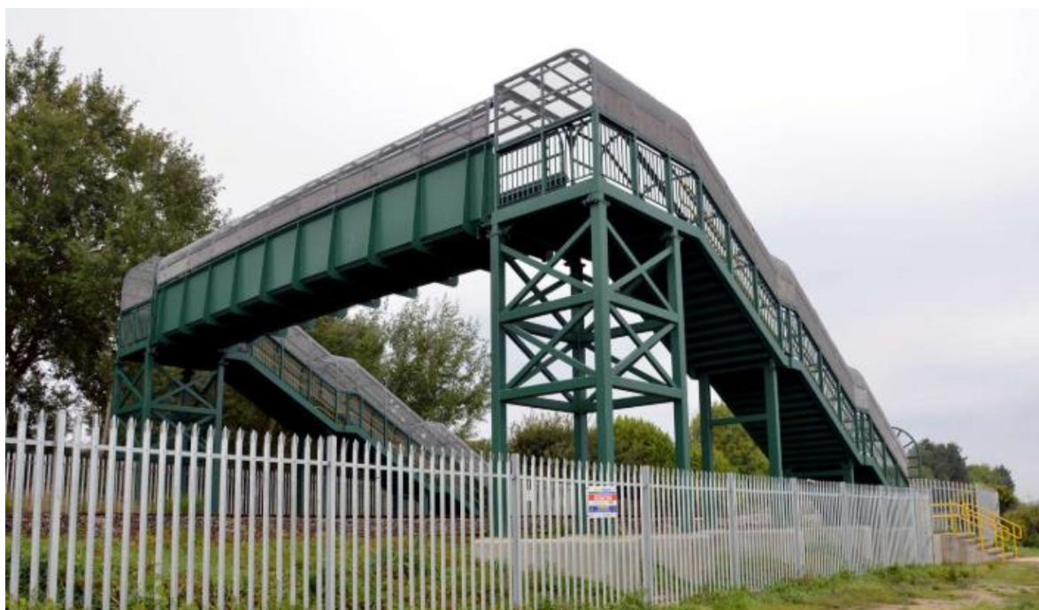
Figure 2-4.3.1 – Typical steel frame support used for pedestrian/cyclist bridge crossing a railway
