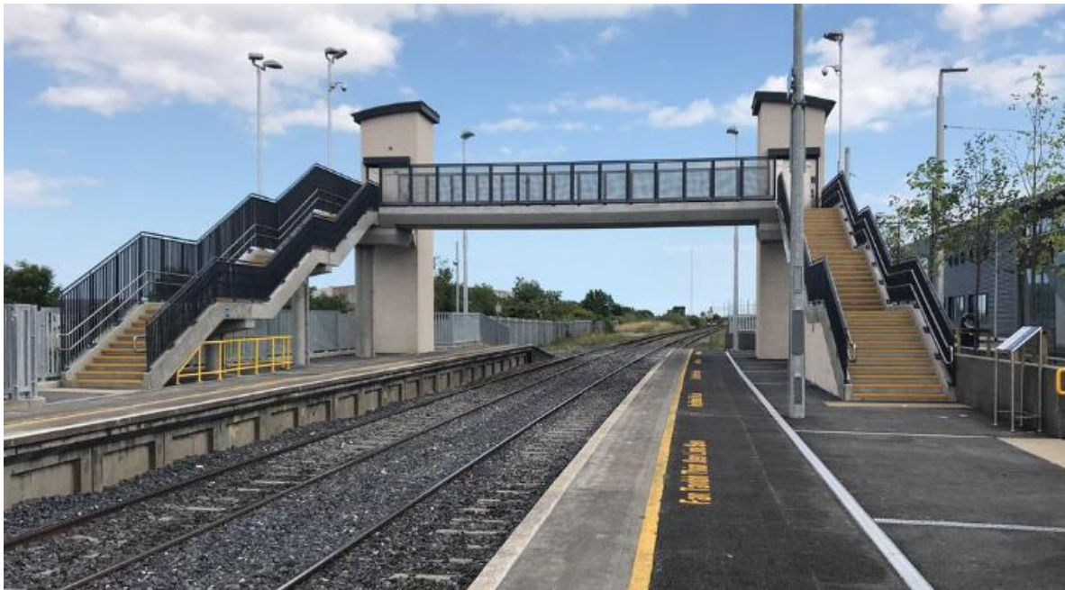
Figure 2-5.2 - Typical Vierendeel Truss crossing a Railway
