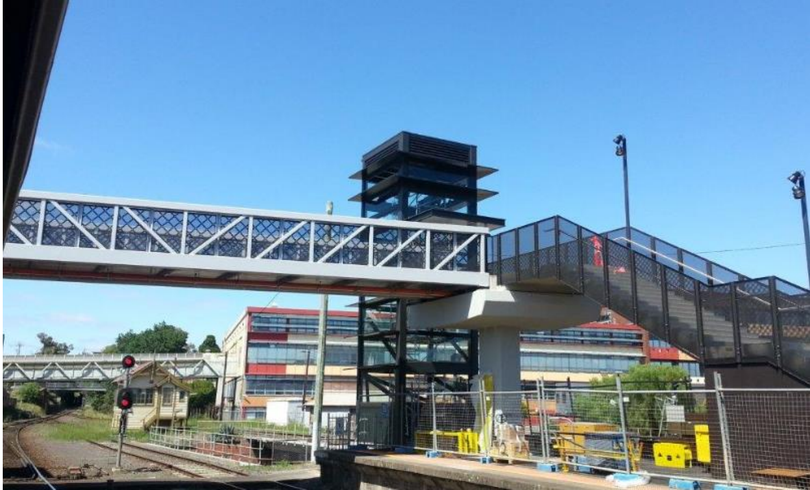
Figure 2-5.1 - Typical Pratt Truss crossing a Railway
