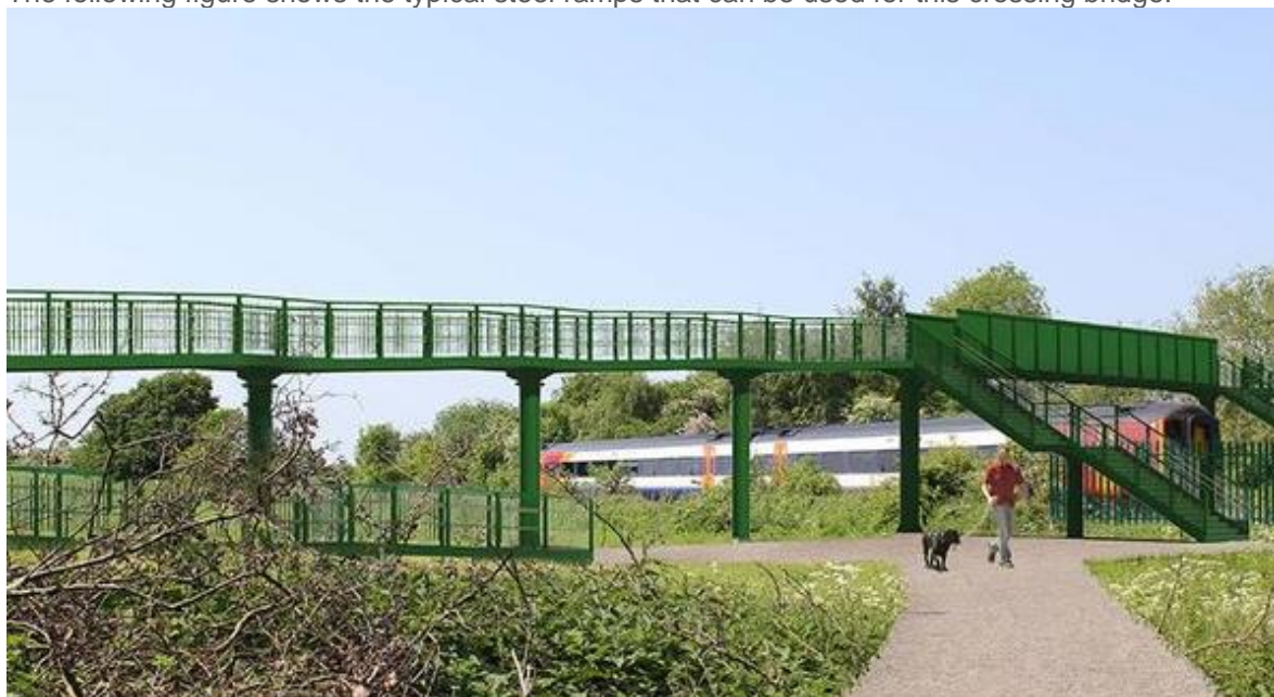
Figure 3-2.1 – Typical steel ramp arrangement
