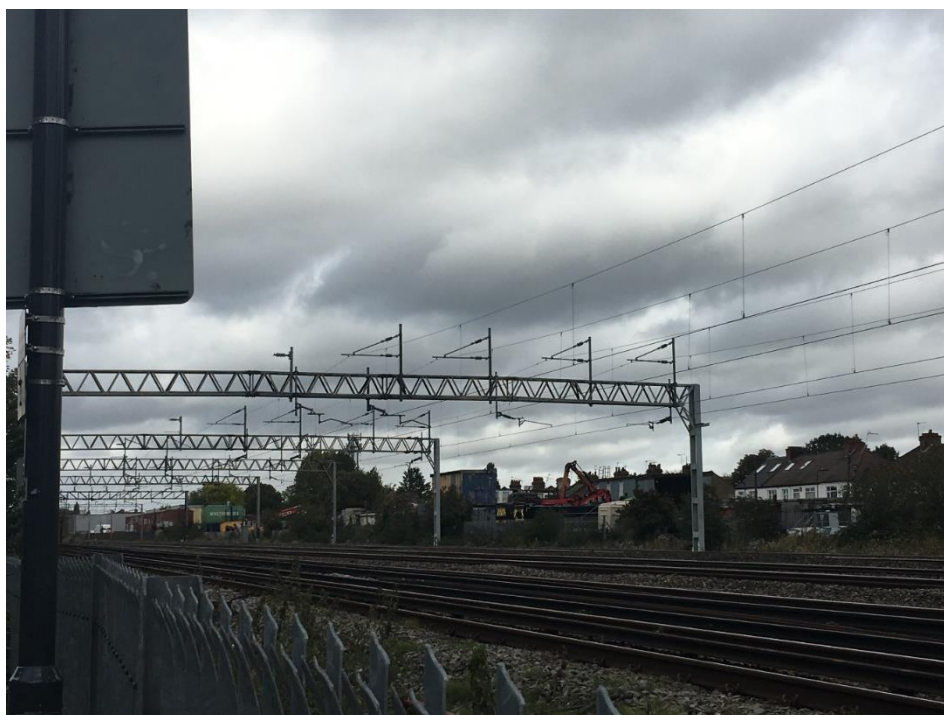
Figure 5-1.1: Photograph showing the OLE system
