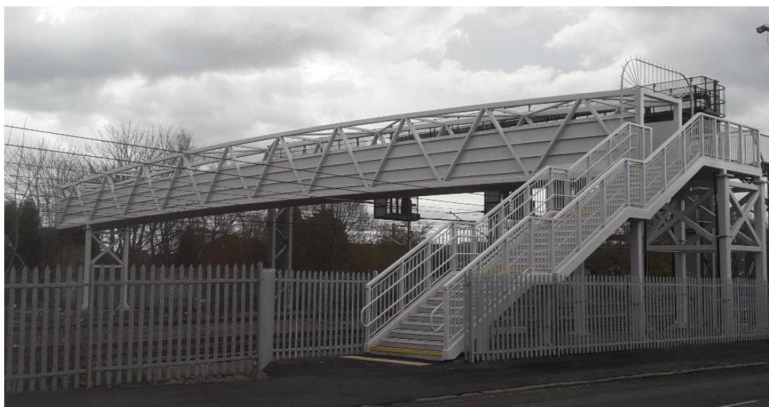
Figure 2 - 4.1.1 – Typical Warren Truss crossing a Railway
