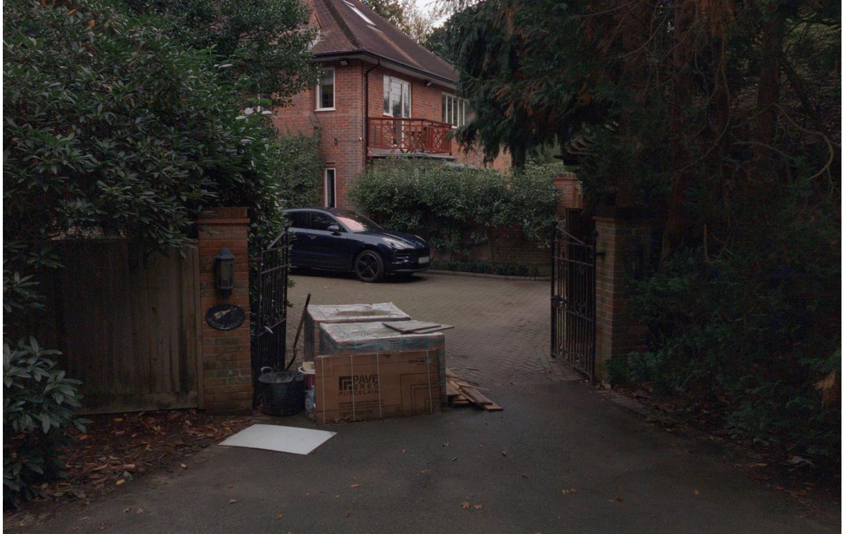
Metal entrance gates at: HeathLodge.
