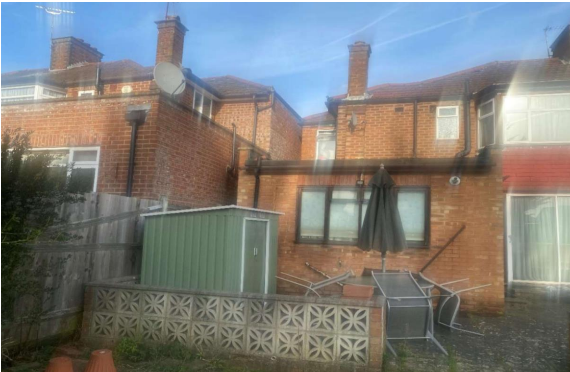
Figure 4: Photograph showing adjoining property at no. 16 Wetheral Drive
