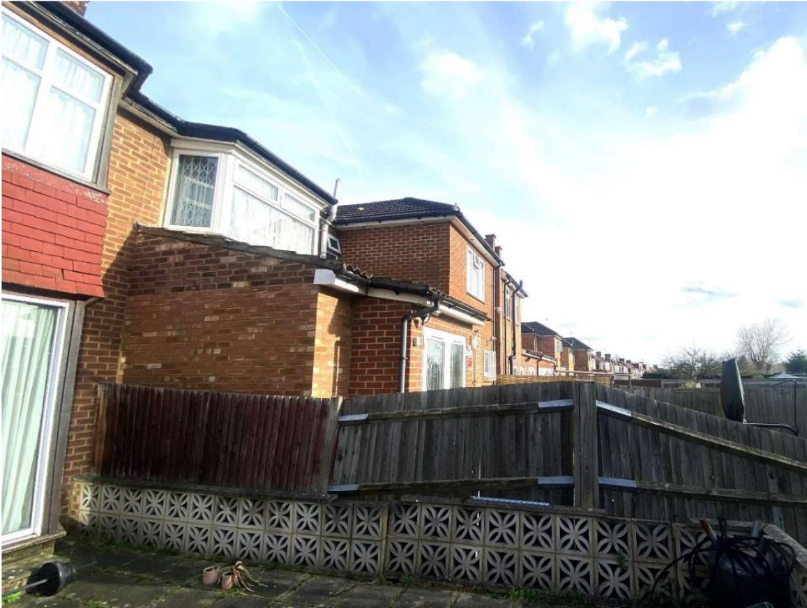
Figure 3: Photograph showing adjoining property at no. 20 Wetheral Drive
