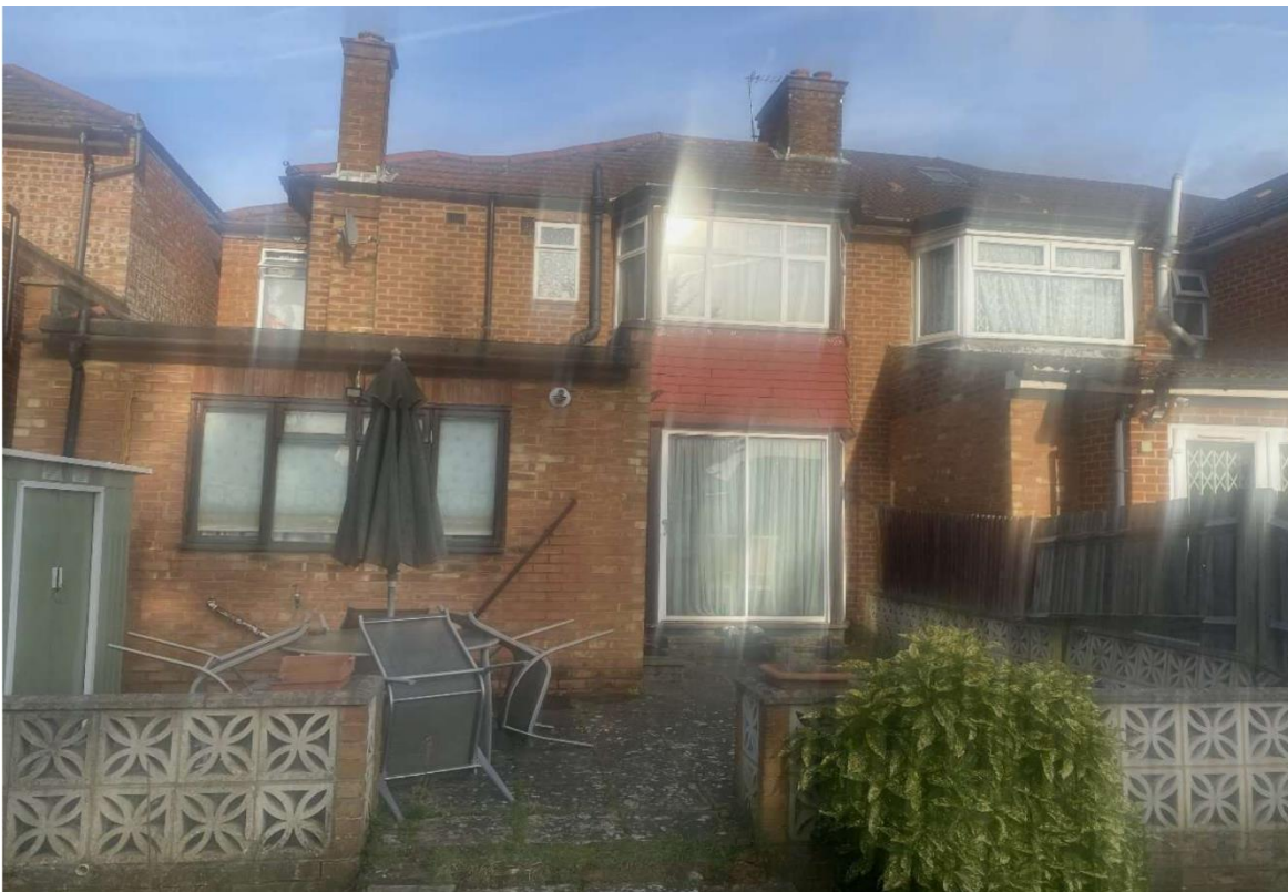
Figure 2: Photograph showing rear of property.
