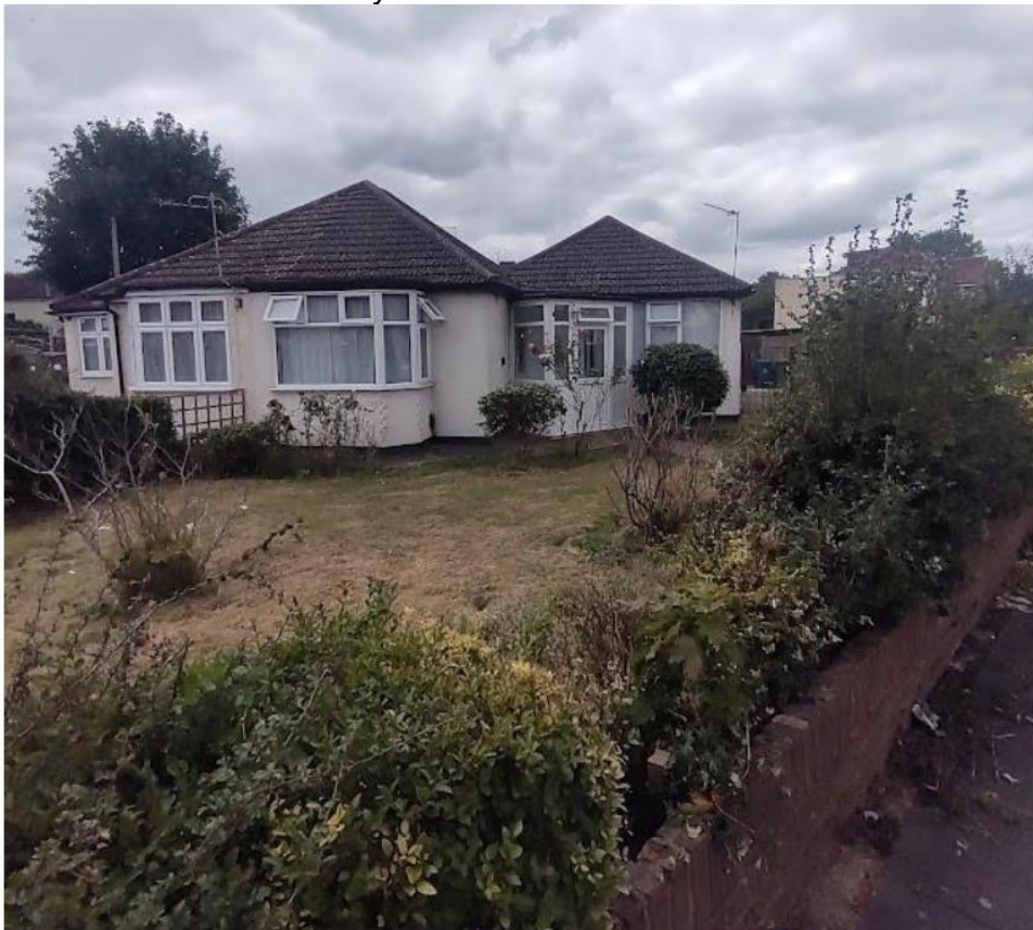
Front Elevation of 1 Carlyon Avenue:
