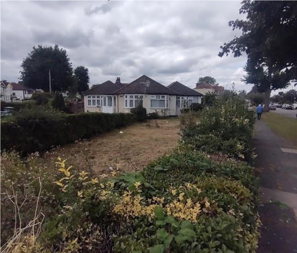
Front Elevation of 1 Carlyon Avenue:
