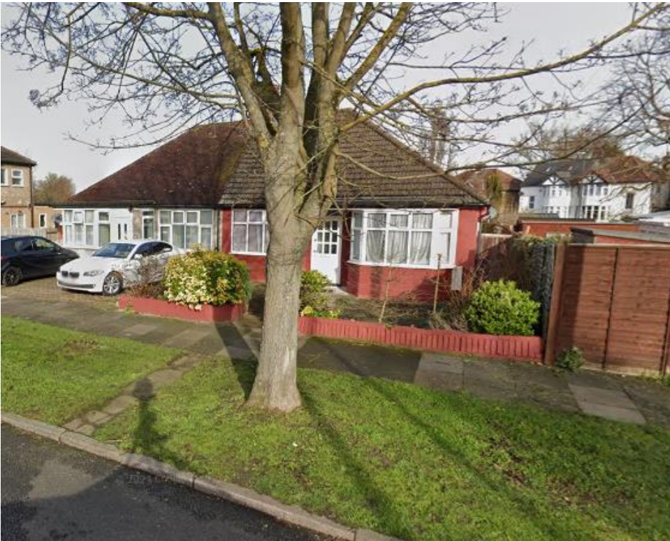
View of 42 and 42A Somervell Road:
