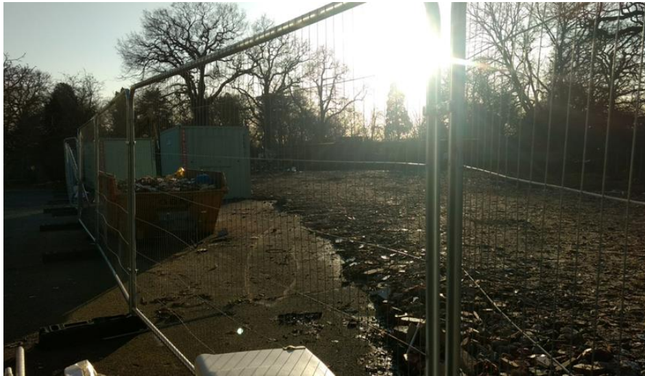
Photo 3 - Within the site facing west
