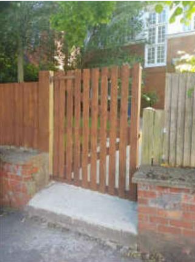
Photo of retrospective gate to be replaced
