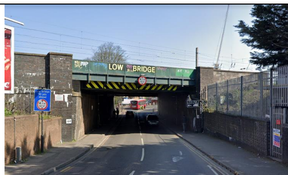
Headstone Drive – Review barrier caused by narrow width at bridge – possible one way shuttle signals, use of Kodak s106 funds
