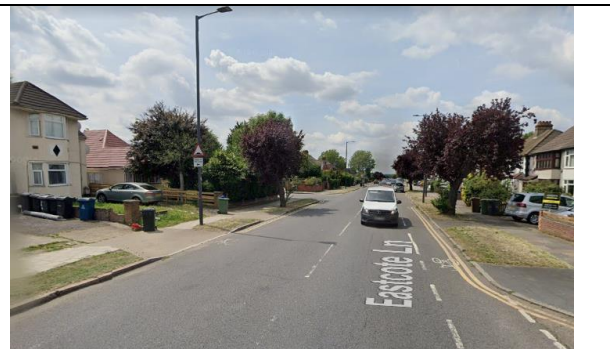
Eastcote Lane – cycle lanes, provide physical segregation, parking controls
