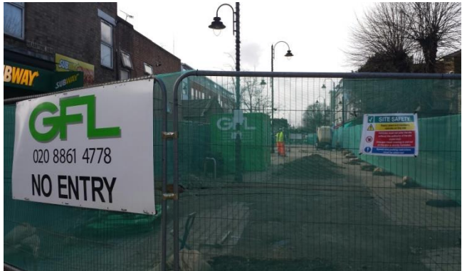
Works at Wealdstone Square
